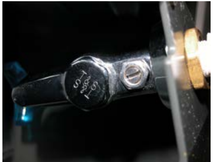
Water Flow Adjustment Screw
