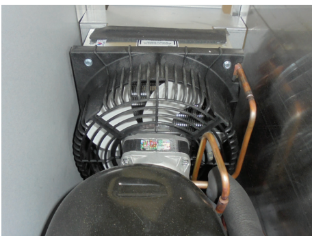
SERVICING THE CONDENSER FAN
