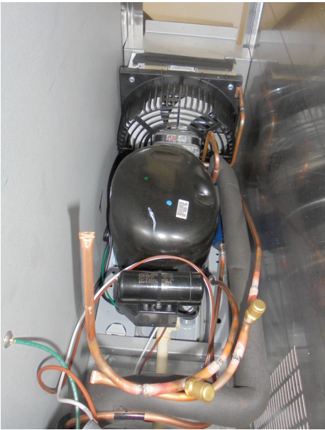
SERVICING THE COMPRESSOR
