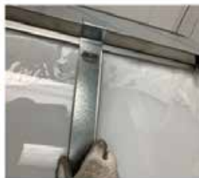
Lid locking bar assembly Place the Lid locking bar as shown above. Make sure the top hinge is aligned and inserted into the slot provide in lid locking bar
