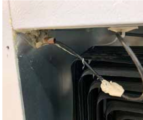
Sensor probe with bulb well foamed
