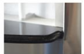
Granite shelf & S/S apron
